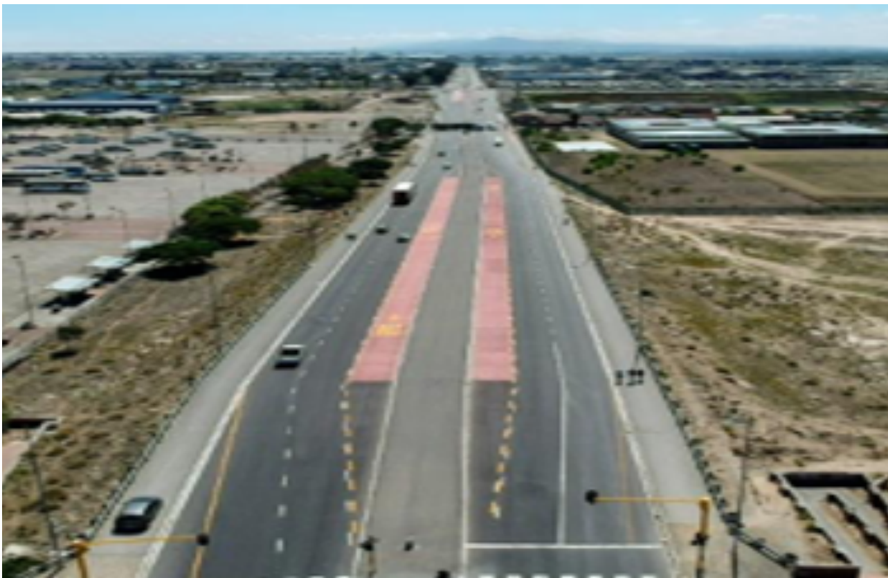
FIGURE 11: The Stock Road dual carriageway completed as part of phase 2A
