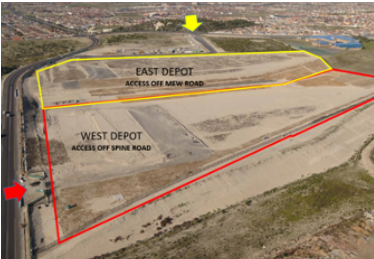
FIGURE 12: The sites for two of the phase 2A bus depots
